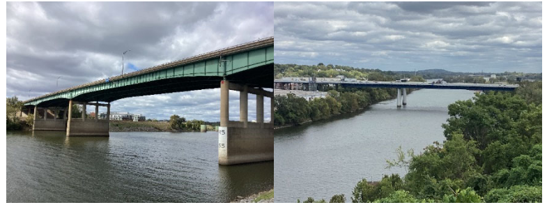
Figure 22 – Interstate bridges over Cumberland River in downtown Nashville
